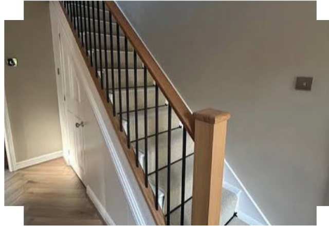
OAK DOORS, HANDRAIL, BASERAIL & NEWEL POST TO STAIRCASE
